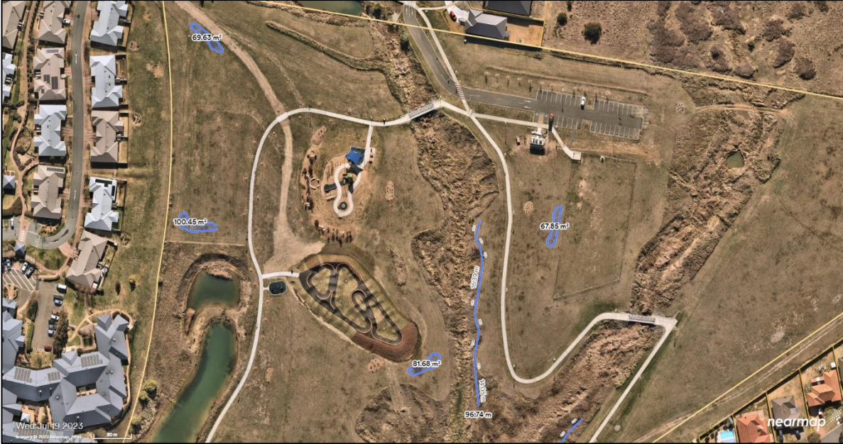
Proposed tree plantings to riparian corridors and the four raised beds to the northern parts of Riverside Park.
